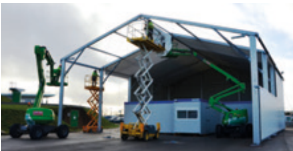
Installation du hangar.
